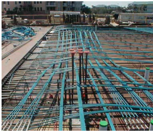
High tension cables prior to the concrete being poured.
