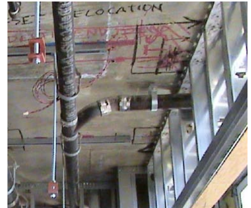
Concrete ceiling with markings indicating where the GPR detected obstructions.
